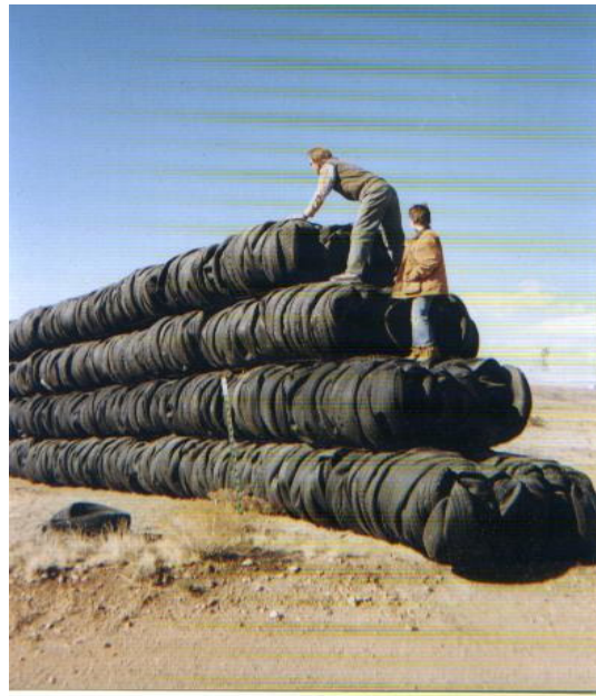
Figure 4 – Four-High Bale Wall
