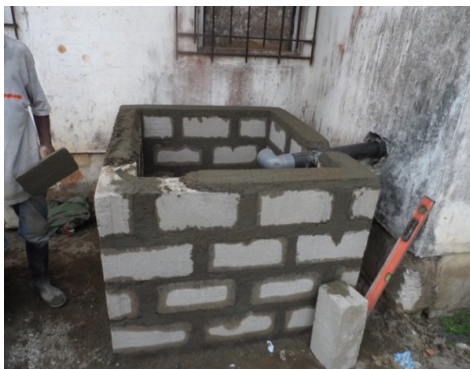
Figure 14: Construction of an above-ground biodigester.
