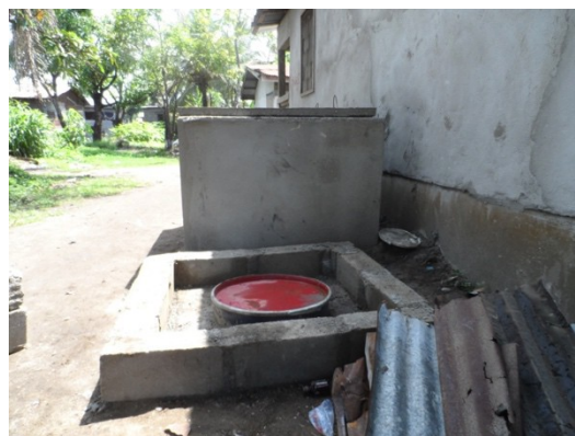
Figure 22: An effluent collector constructed with a plastic drum in Liberia. Protection walls have been raised around the drum to protect it against flooding.
