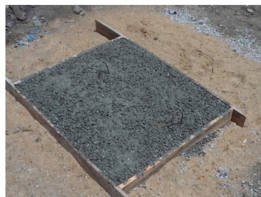
Figure 19: Precast reinforced porous slab, Liberia.
