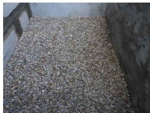
Figure 17: Set-up of the upper layer of the drainage layer, i.e. 10 cm of gravel, Liberia.
