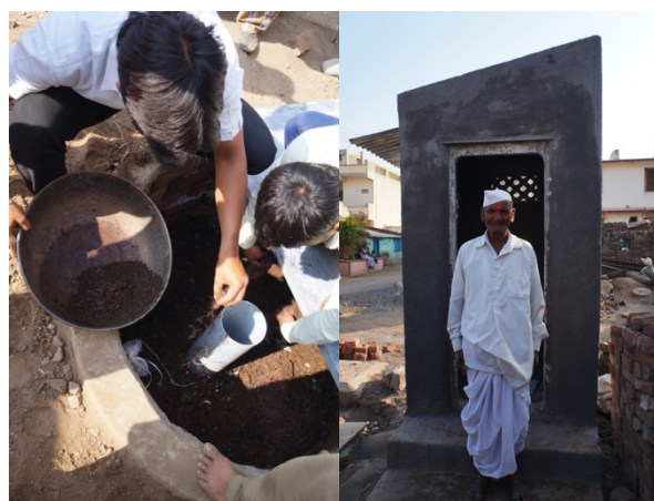
Figure 24: Addition of the worms to the biodigester, India (left). A toilet with its owner, India (right) [23].
