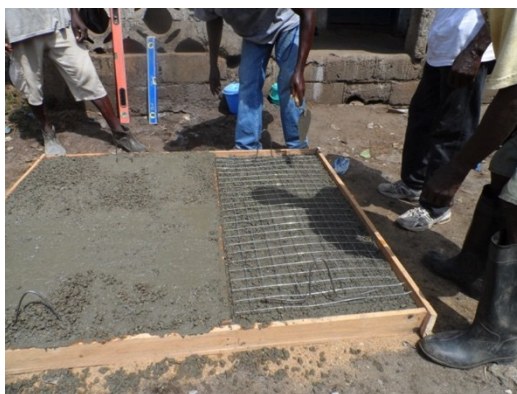
Figure 15: Pouring of a cover slab, Liberia.
