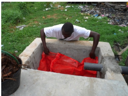
Figure 20: Positioning of onion bags above the drainage layer, Liberia.
