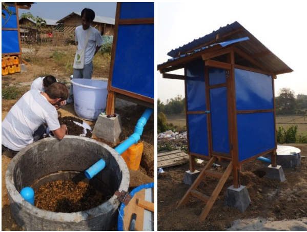
Figure 25: TWTs installed in the Maina IDPs camp in Myanmar [24].
