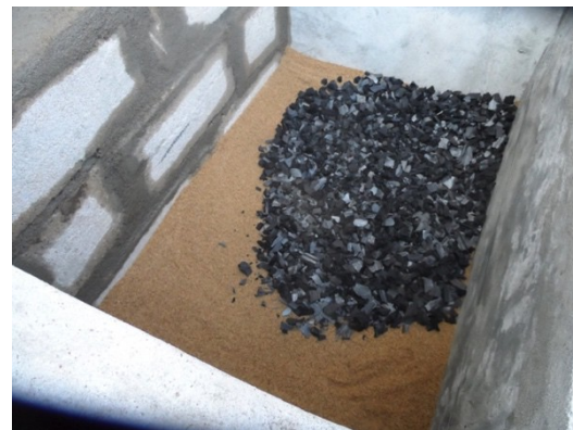
Figure 16: Set-up of the bottom layer and the intermediate layer of the drainage layer, i.e. 15 cm of sand and 5 cm of charcoal, Liberia.
