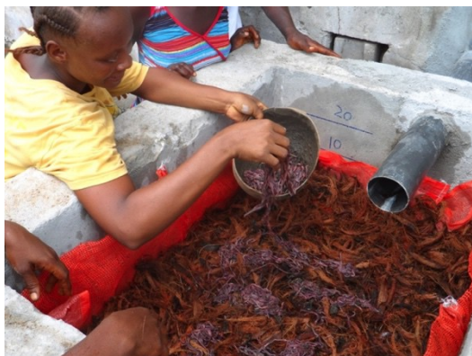
Figure 21: Provision of worms to the biodigester.
