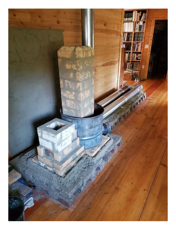
Mixing the cob was the most labor intensive part of the job, but it was rewarding. Here, most of the cobbing was complete. Notice the location of the clean outs for the manifold and the channel.
