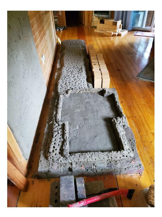
This is the completed core. The mortar is clay slip. The firebrick is rated 3000F. I used hardened bricks for the wood feed in order to be more durable when feeding the fire. These bricks are lighter in color and were more expensive. I used 10 of these.
