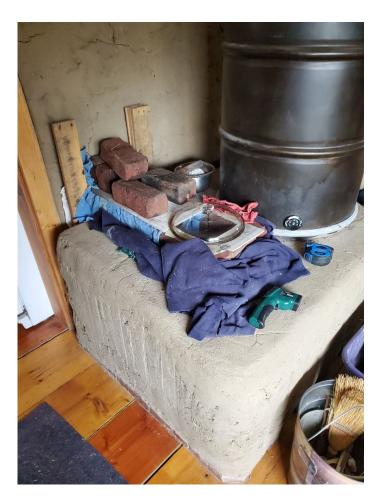
The second cold air draw I am planning will be a draw channel that will run horizontally from behind the vertical flue near the floor directly to the manifold that is presently buried inside the cob, then upward next to the manifold through an oblong shape vertical cob flue. I will have to take out some cob to implement this feature and build up a cob flue that will rise to the height where the manifold meets the bottom of the barrel.
