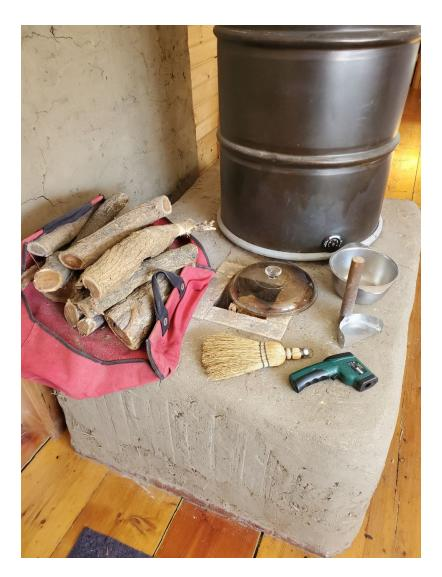
The stainless steel bowl was used to haul out ashes. I usually filled it up after 2-3 burns. The homemade scraper worked great to scoop the ashes out of the burn tunnel.
