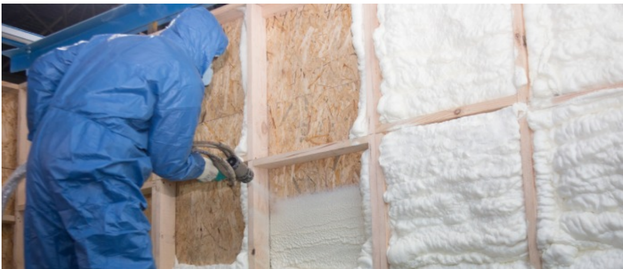
Applying closed-cell spray foam on interior walls. Typical R-value is R-6 per inch.
