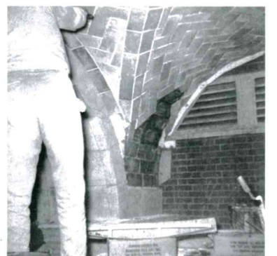
Fig. 4.26 Adding final layer of Guastavino tile on underside of vault, National Shrine of the Immaculate Conception, Washington DC, 1958
