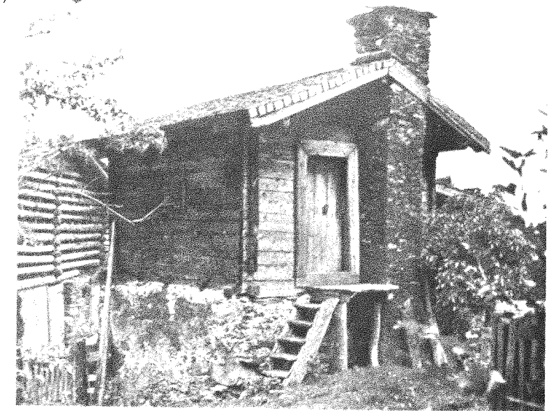
Figs 396 and 397 Two modest log cottages, built as accommodation for retired farm people (Hofgastein, Austria). In both cases, the chimney is built so as to be independent of the settling of the log walls.
