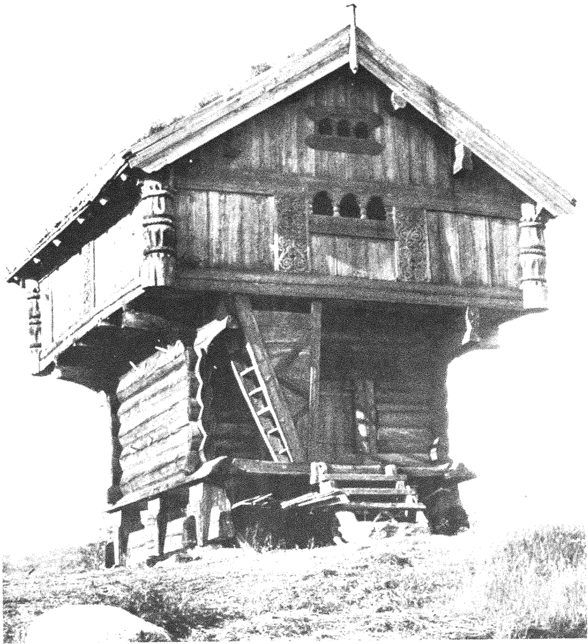
Fig 388 Stabur from Telemark. A beautiful example of the extensive use of grooved or moulded edgework, at times even run onto the end grain.
